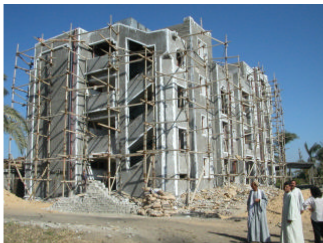
NSP-funded primary school under construction in village
