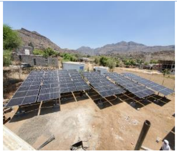
Supply and installation of solar pumping system by capacity 69 KW for Al Nashamah Water scheme, Al Nashamah area - Al Sawaa sub-district - Al Ma'afer district, Taiz'z Gov.
