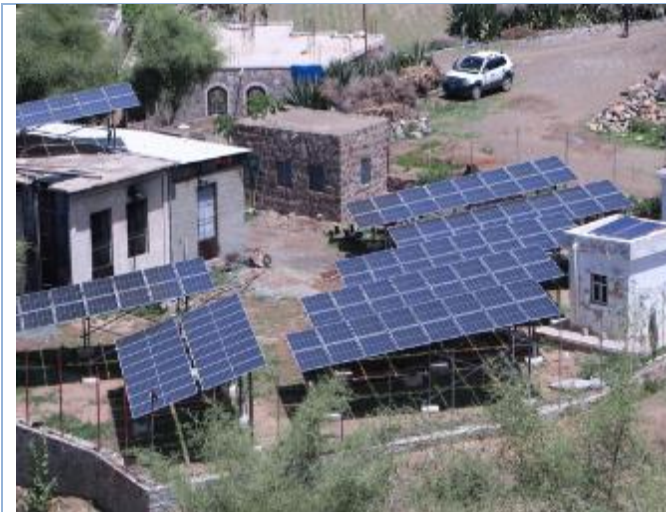
Supply and installation of solar pumping system by capacity 69 KW for Al Nashamah Water scheme, Al Nashamah area - Al Sawaa sub-district - Al Ma'afer district, Taiz'z Gov.
