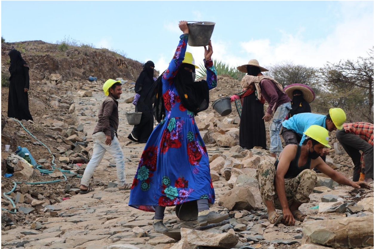
Image 2 – Fatima and other villagers rehabilitating the road to their village
