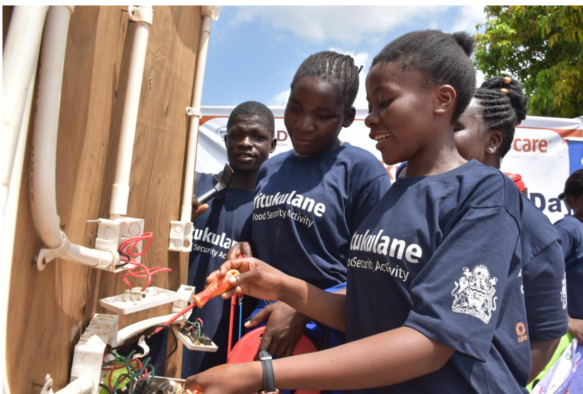
Titukulane youth in Zomba trained in electrical installation © Titukulane 2023 / Samuel Chibaya
