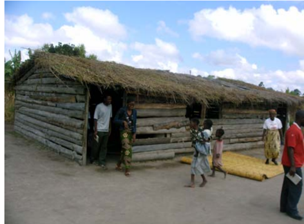
CBCC structure built by the community at Mbawemi FBO in Mzimba– 30/05/2008
