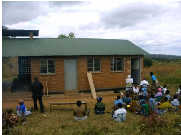
Rehabilitated VCT centre at Kapelula in Kasungu by WVM – 28/05/2008
